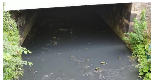
▲ Bradford Beck, downstream of George Street tank
